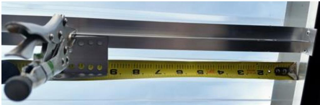
7. Clamp the Frame Bracket in place to either the Ridge (1000 series) or the Hanger bar T-Bracket (all other series) starting at **9" from the gable end**. The thin side of the bracket points to the gable end.
